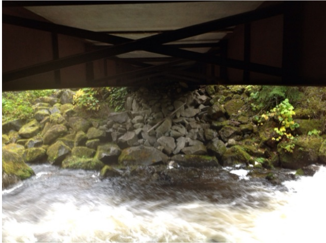
Right Bank Abutment when facing downstream
