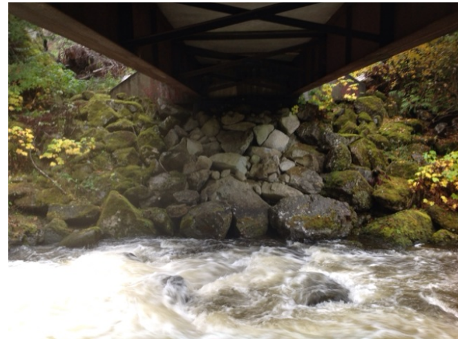
Left Bank Abutment when facing downstream
